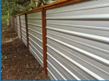
Boundary Wall Metal Sheet
