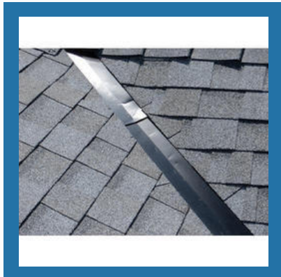
Metal Roof Flashing
